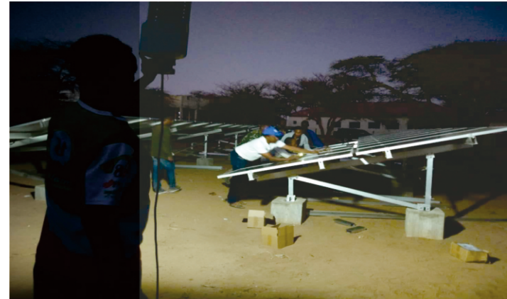
Birjeex Camp: 20KW Solar Off Grid System
